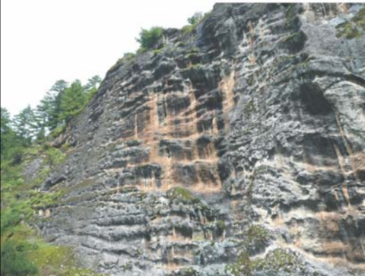
Fig 5. Light erosion strips, cliff No. 7.
